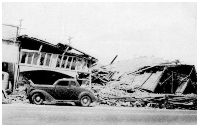
Fig. 1.2 Collapsed buildings in Imperial, California, after the May 18, 1940 El Centro earthquake. (U.S. Coast and Geodetic Survey photograph)
