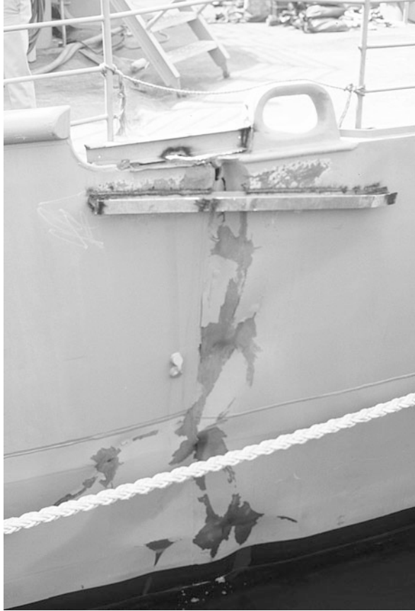
Fig. 9.27 Photograph of USS Princeton's cracked hull after and the temporary at-sea patch following the 1991 sea mine incident (U.S. Navy photograph)
